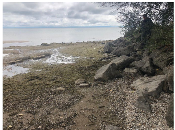
Photo 11: Western limit of beach at constructed berm
