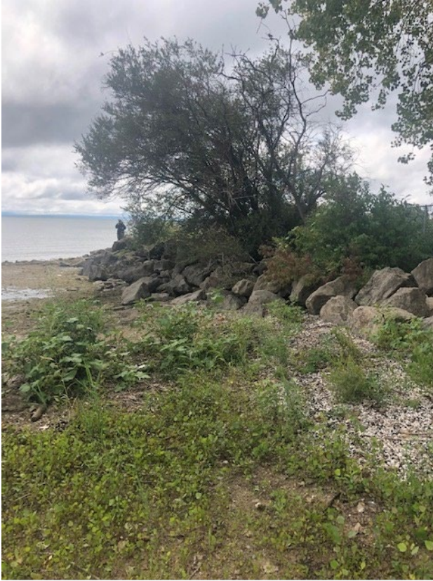
Photo 14: Extent of earthen berm and rocks at base of fence
