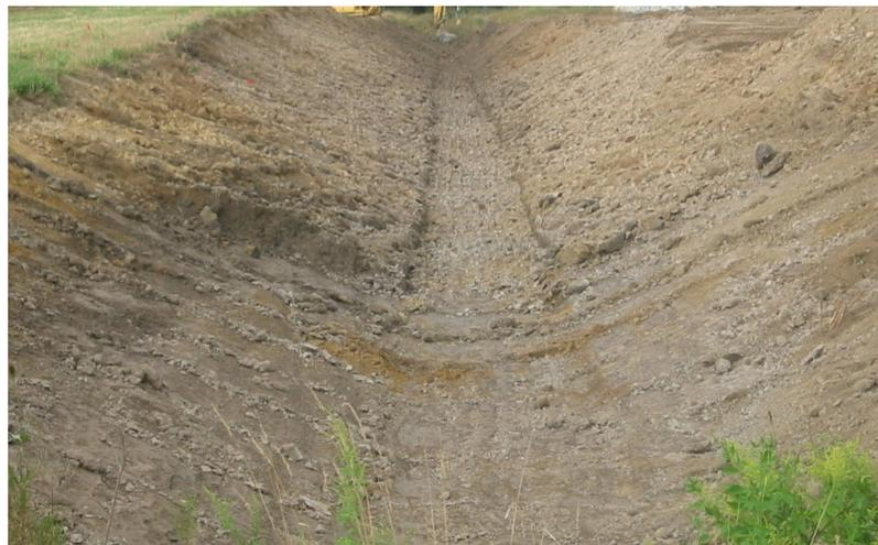
**Figure 12 Trapezoidal Ditching Under Construction**
