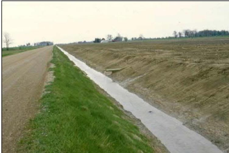
**Figure 8 Example of clear drain**
