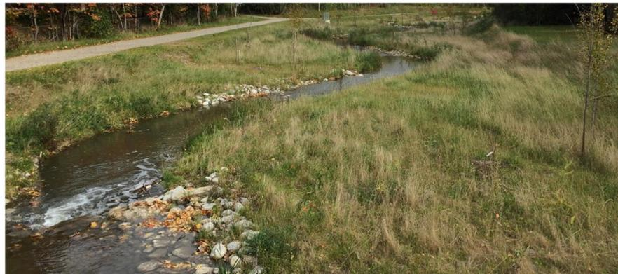
**Figure 14 Naturalized Channel with Pools and Riffles**
