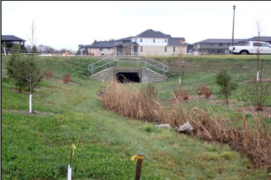
Photograph 1. Example of Wing Culvert Design for Road Crossing of a Watercourse and 30 m Wide Naturalized Corridor
