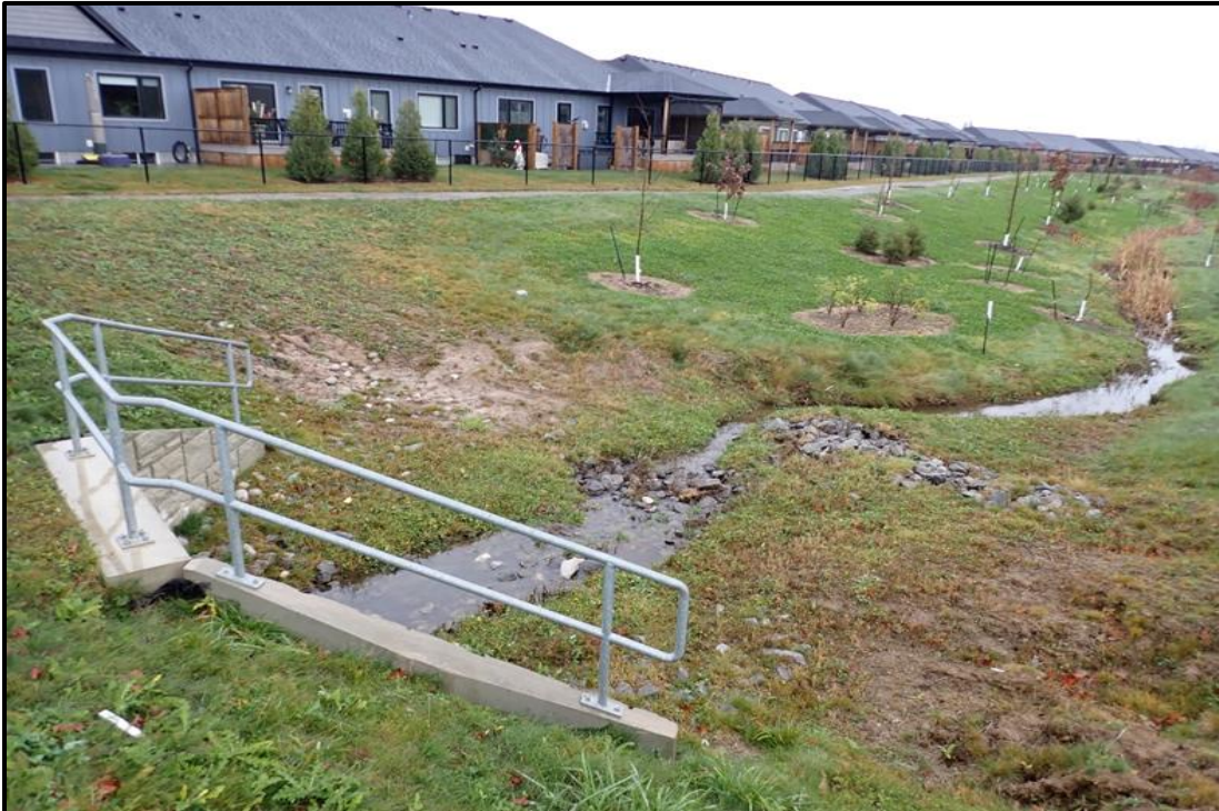
Photograph 3. Example of Wing Culvert Design for Road Crossing of a Watercourse and 30 m Wide Naturalized Corridor
