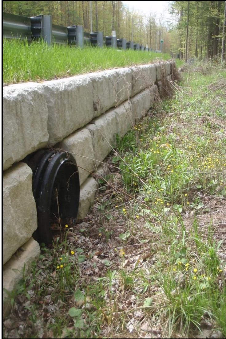
Photograph 7. Example of Road Crossing Barrier to Funnel Reptiles and Amphibians Movements in Corridor
