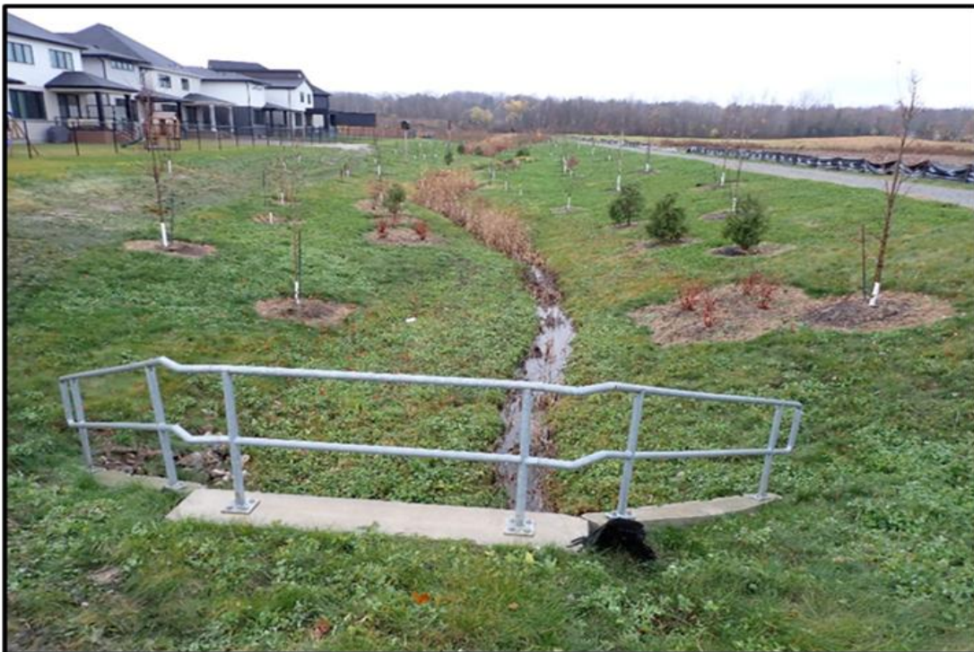
Photograph 2. Example of Wing Culvert Design for Road Crossing of a Watercourse and 30 m Wide Naturalized Corridor
