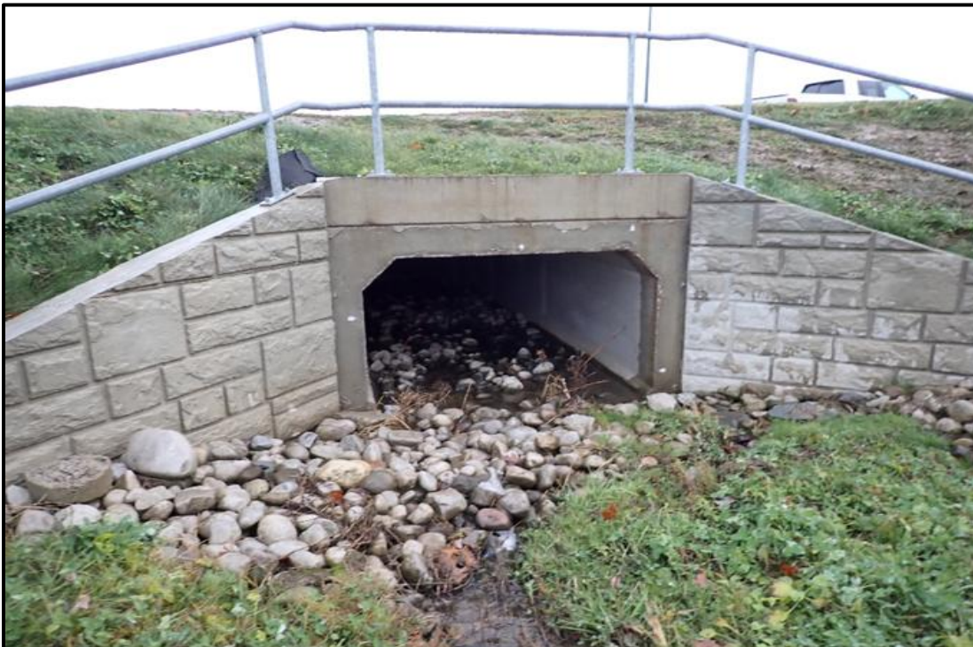
Photograph 4. Substrate Placed on Culvert Bottom to Promote Wildlife Passage
