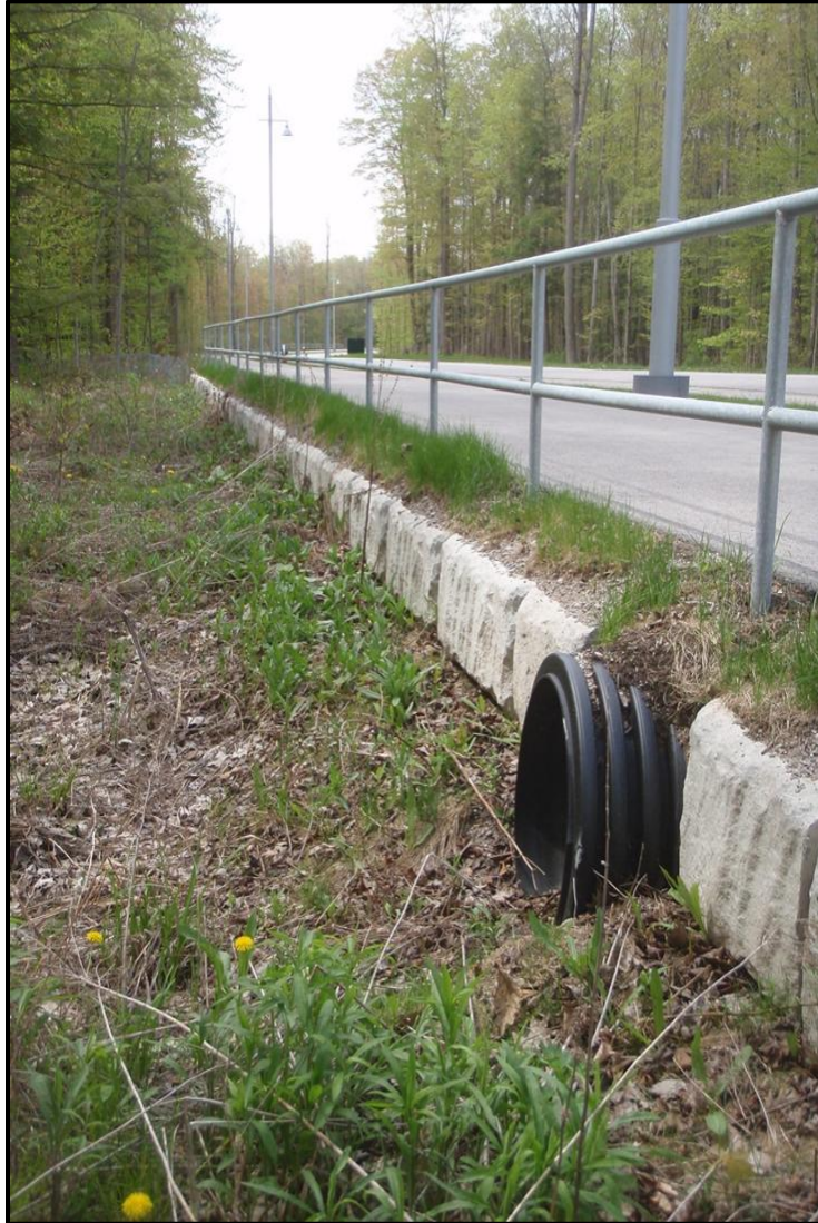
Photograph 6. Example of Road Crossing Barrier to Funnel Reptiles and Amphibians Movements in Corridor
