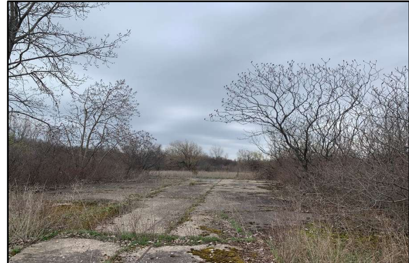
Photo 4. Proposed Area of Disturbance and ground floor slab, facing west (14 April 2026).
