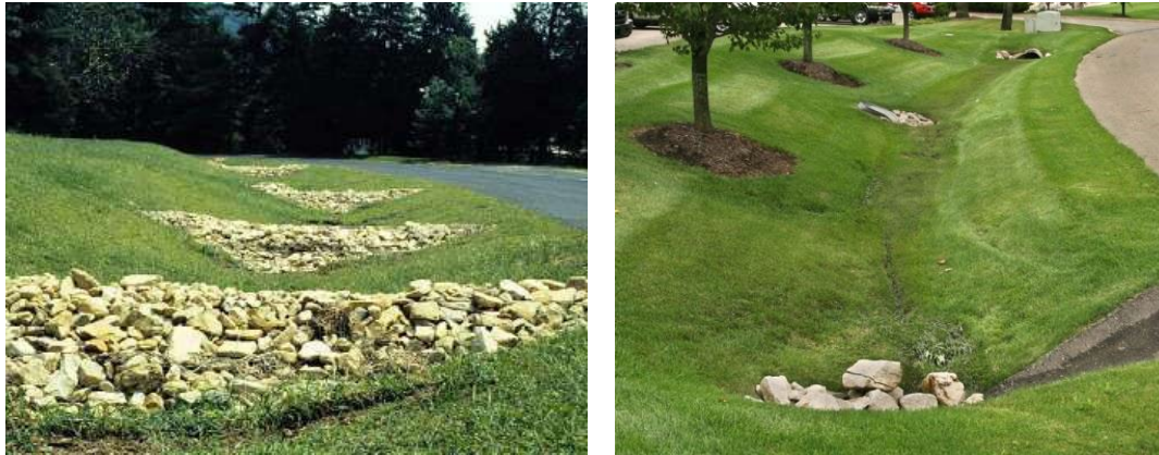
Figure 7 – Sample Grass Swale with Check Dams (LID)
