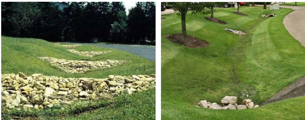
Figure 3 – Sample grass swale with check dams (LID)
