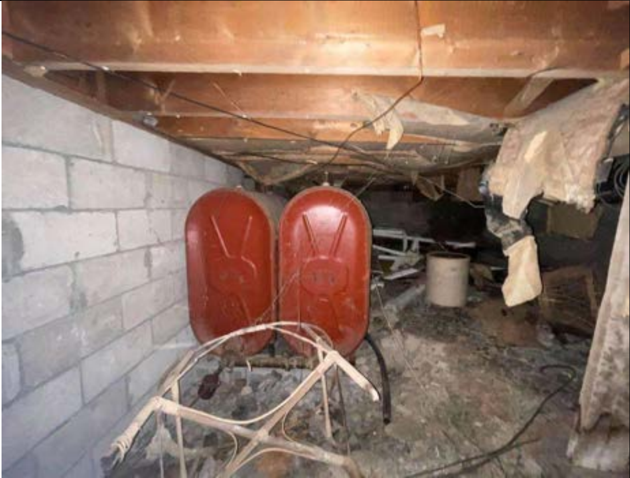
Photograph No. 10 – Two additional ASTs identified in basement crawl space.
