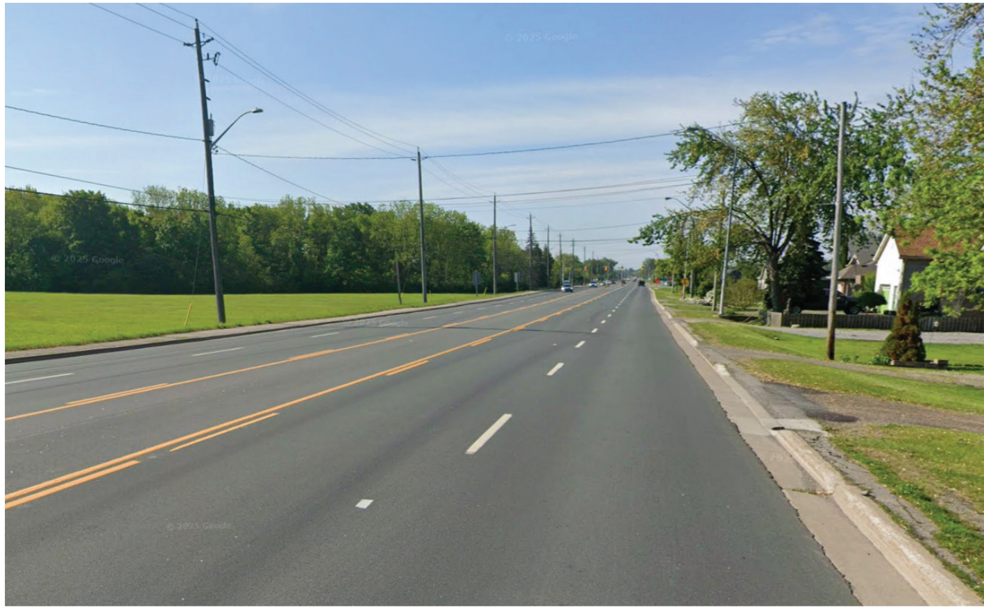
5 View South along West Side Road
