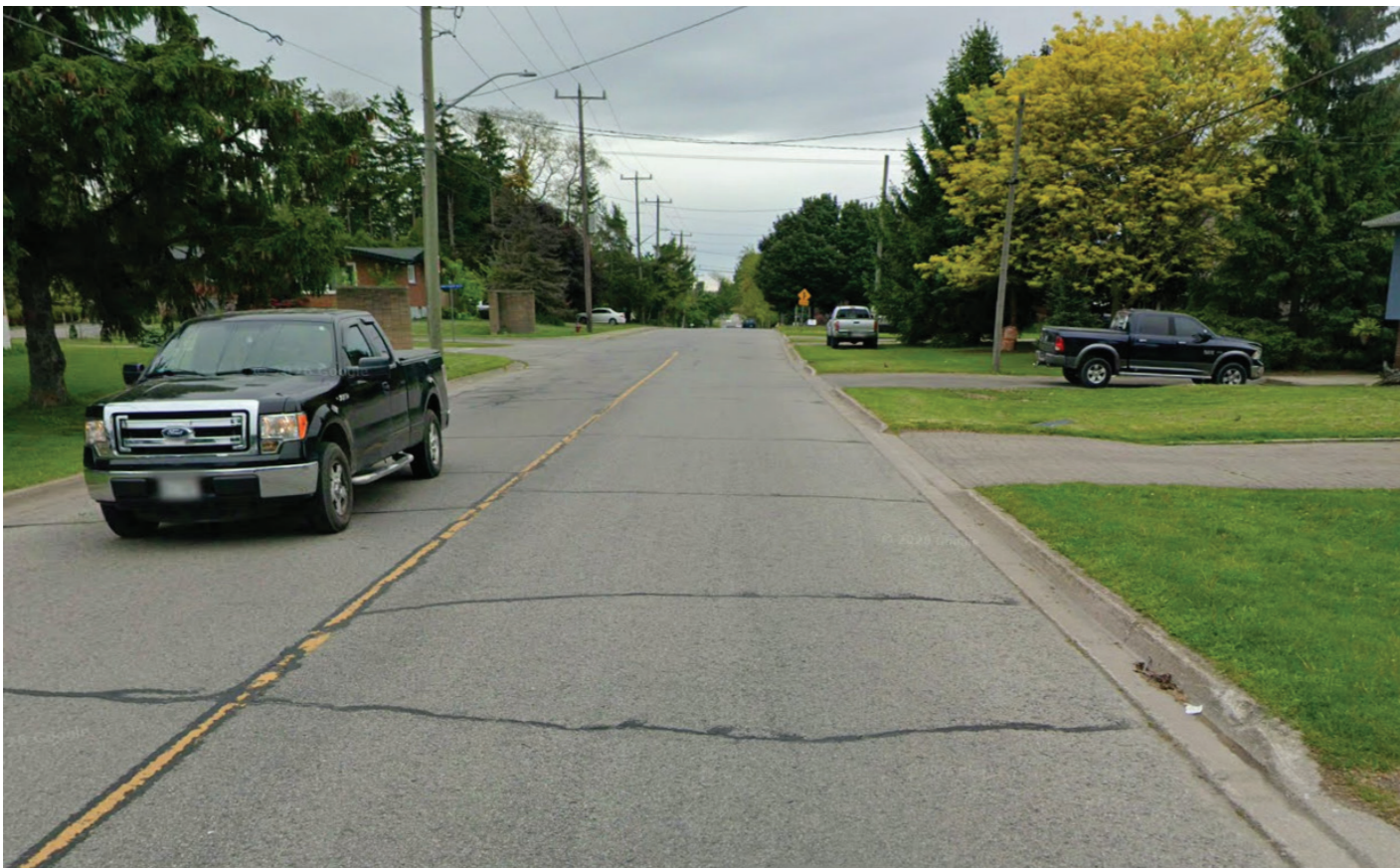
3 View East along Barrick Road (At Secondary Entrance of Subject Site)
