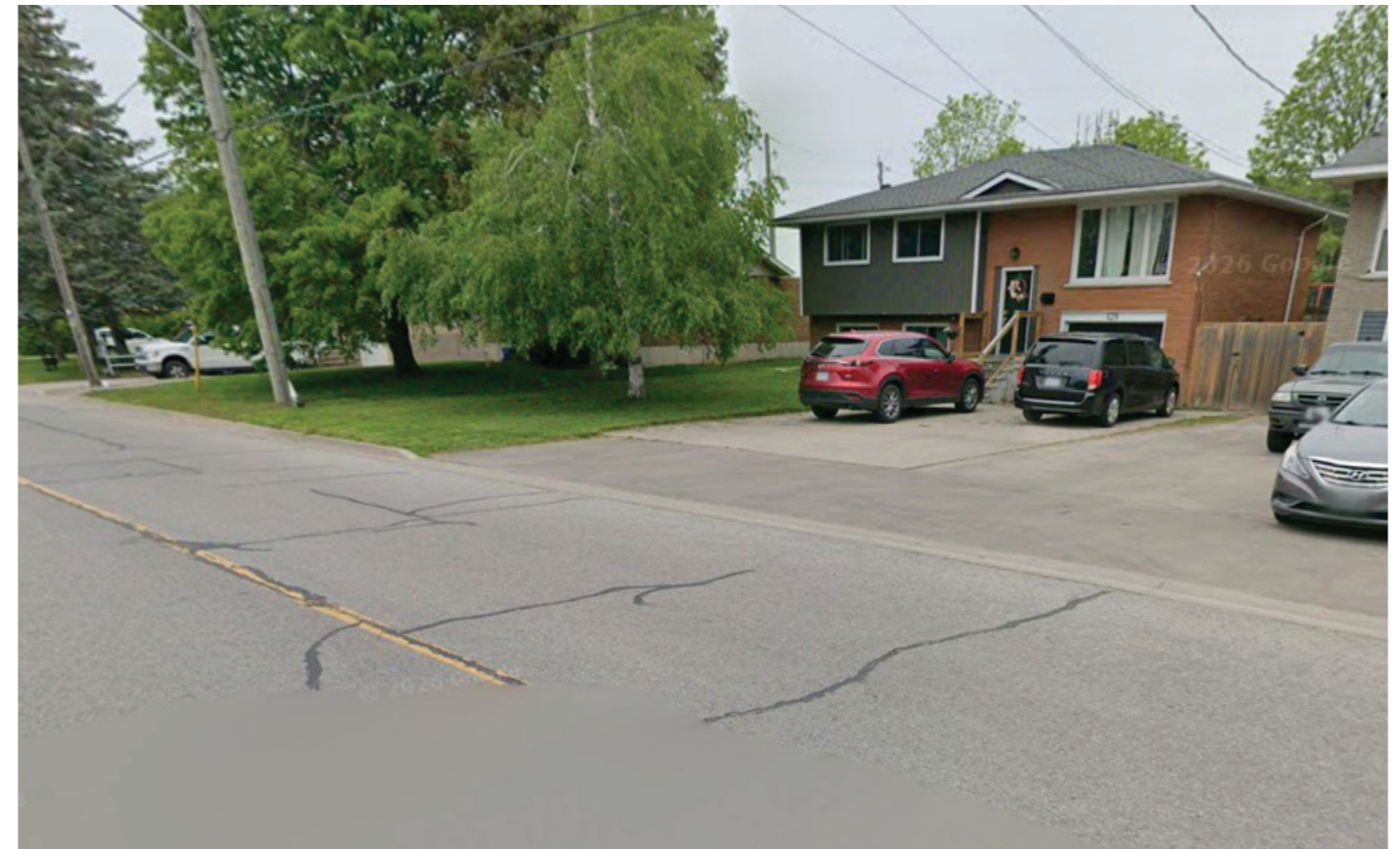
2 View West along Barrick Road (At Secondary Entrance of Subject Site)
