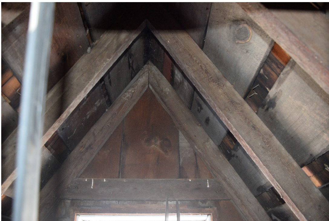
FIGURE 50: DIMENSIONAL LUMBER FRAMING AND ROUGH-CUT PLANK DECKING OF CENTER DORMER OF OUTBUILDING, FACING NORTH
