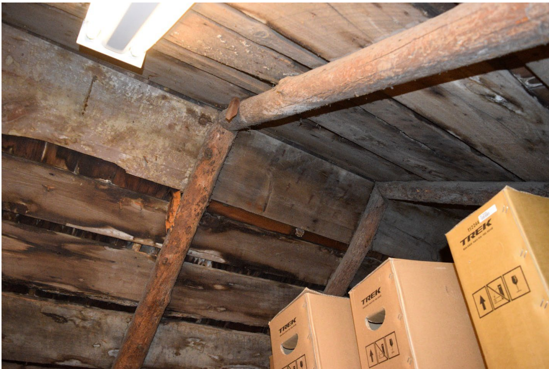
FIGURE 49: TYPICAL EXAMPLE OF ROOF FRAMING USING IN THE ROUND TREES AND ROUGH CUT PLANK SKIN OF OUTBUILDING
