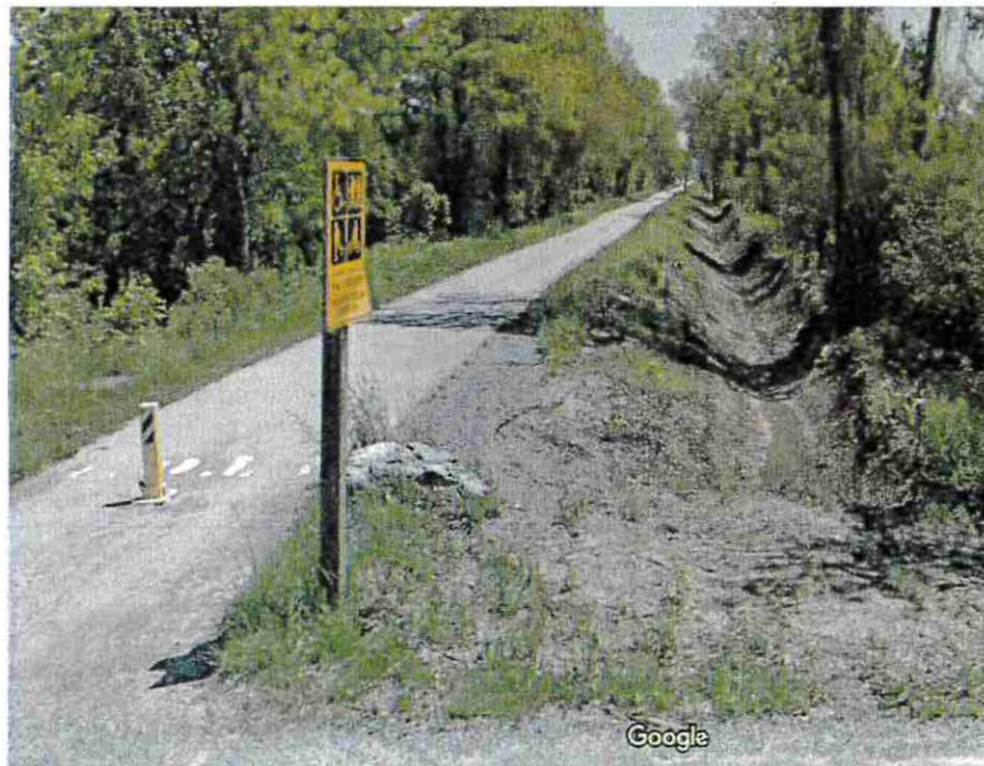
Figure 12 Zavitz West Trail Branch Drain post construction looking East
