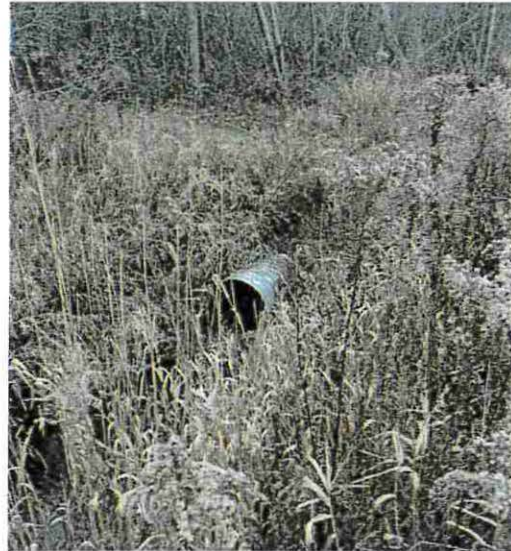
Figure 1 Clee Crossing Culvert looking South
