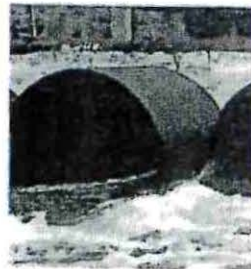
Figure 4-36 Pipe-arch culvert
