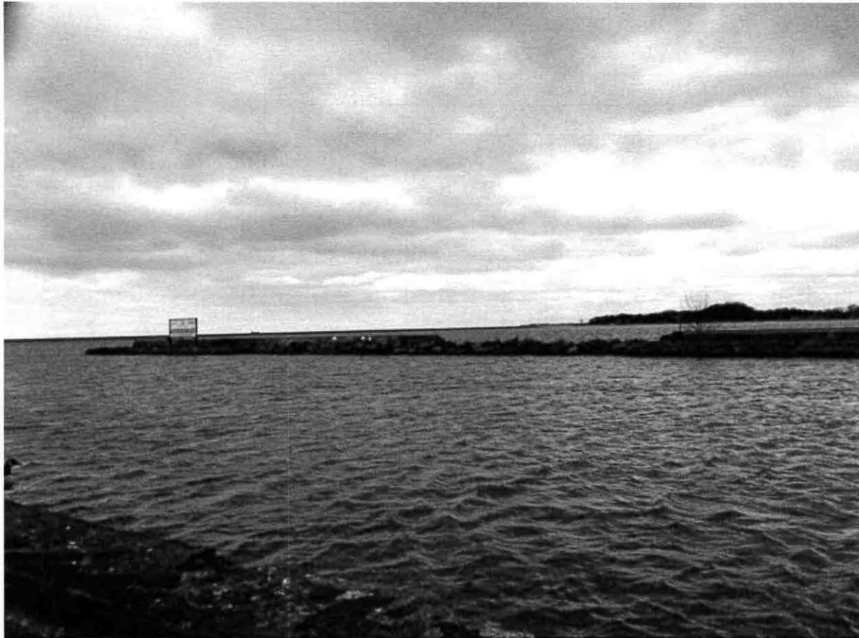
South end of Quarantine Wall
